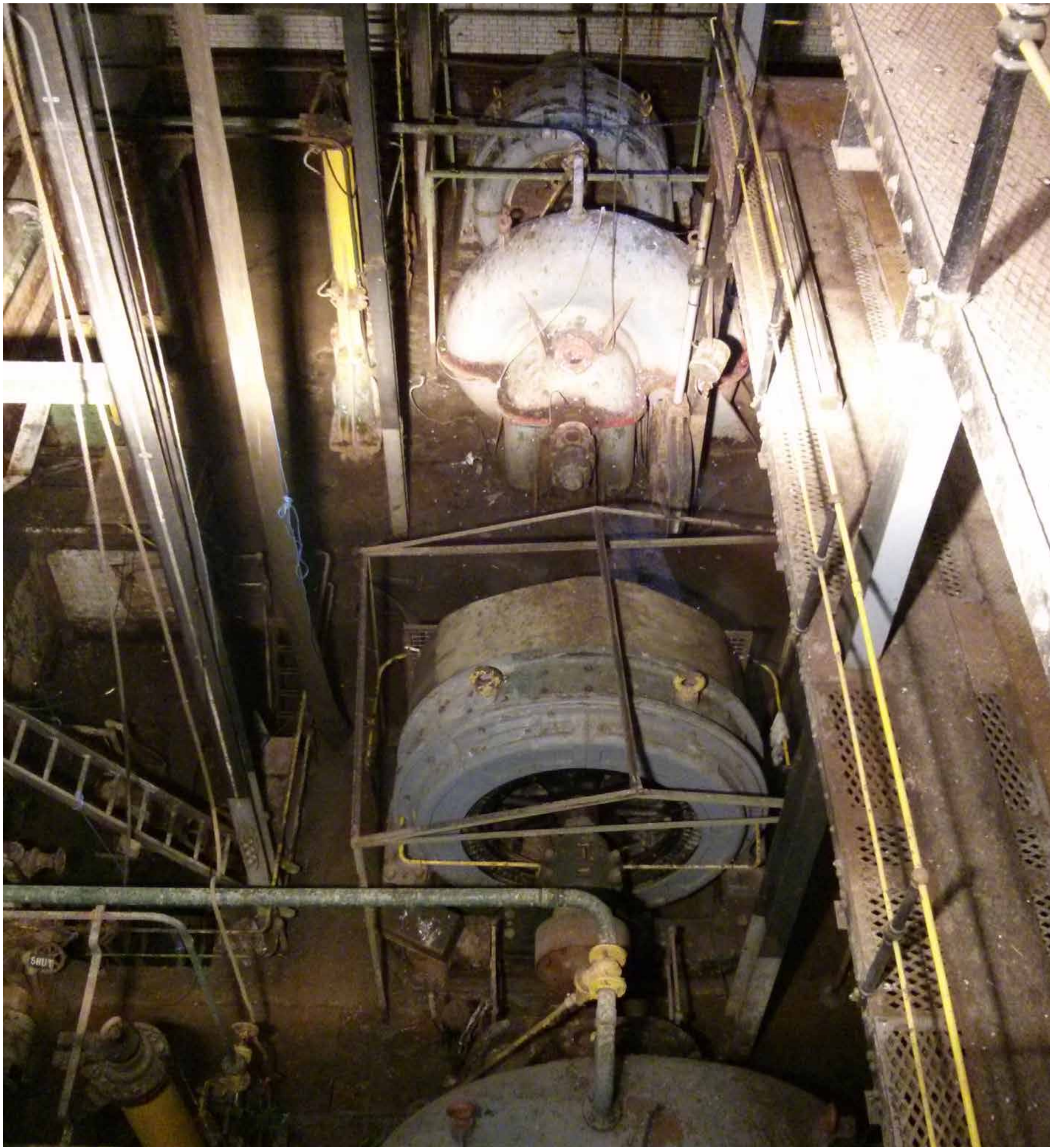
Pump well at Trafalgar Dock
